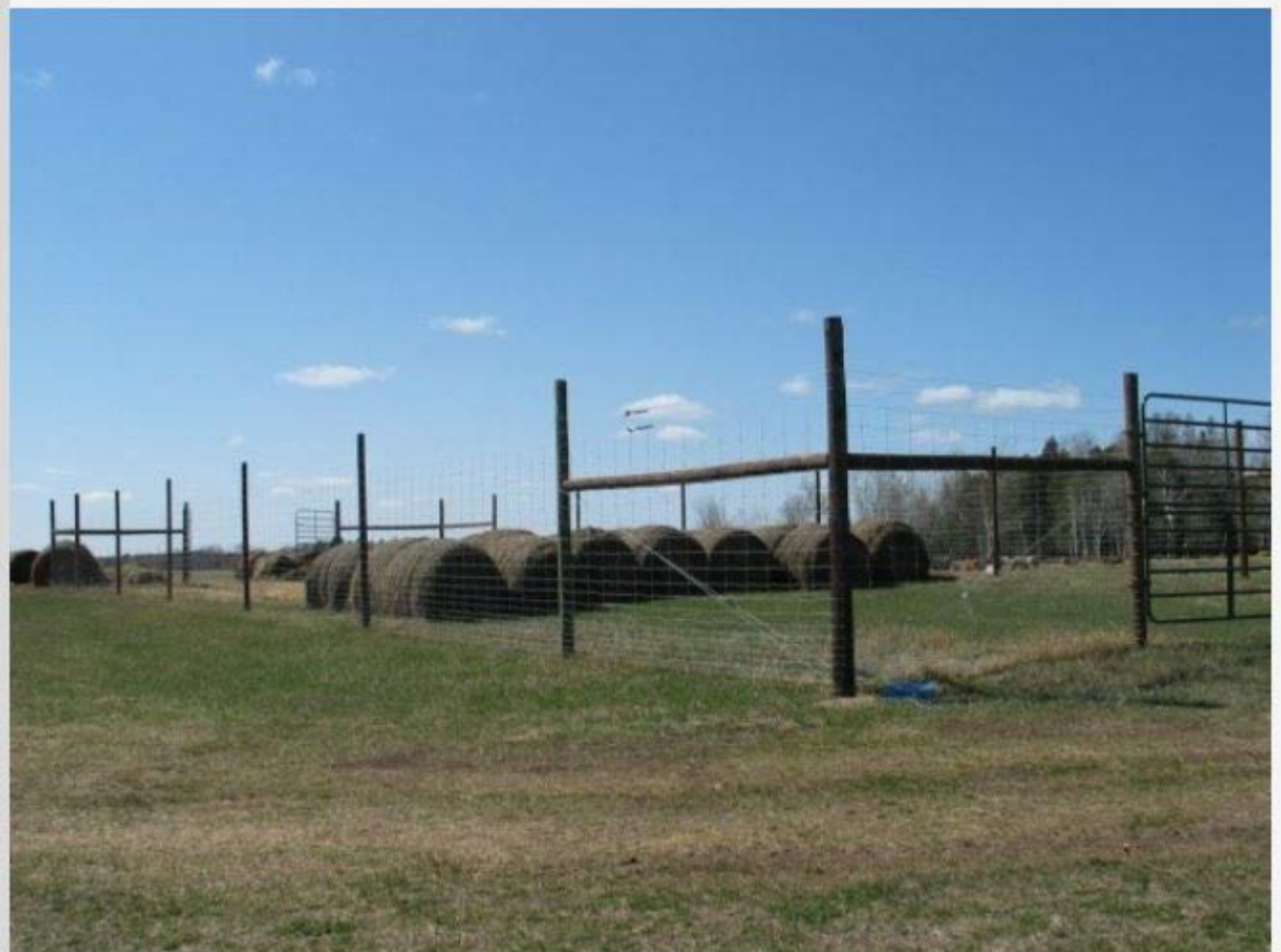
Permanent barrier fence: 10 ft. tall, high tensile woven wire fencing.
