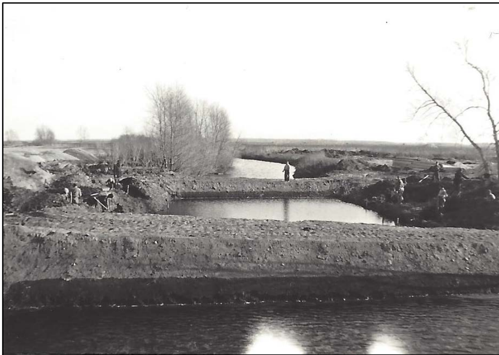
Coffer dam for construction of Haraldson dam, 1937
