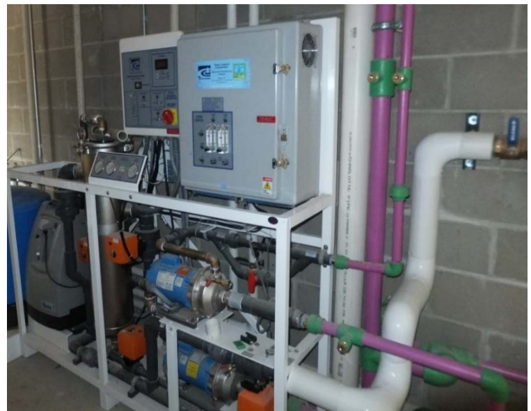
Figure 25. The purple pipes indicate reuse water. A Plumbing Board variance is required for indoor water reuse other than non-potable rainwater catchment systems. This reuse system is located at the new Vermillion State Park sanitation building and is used for toilet flushing.
