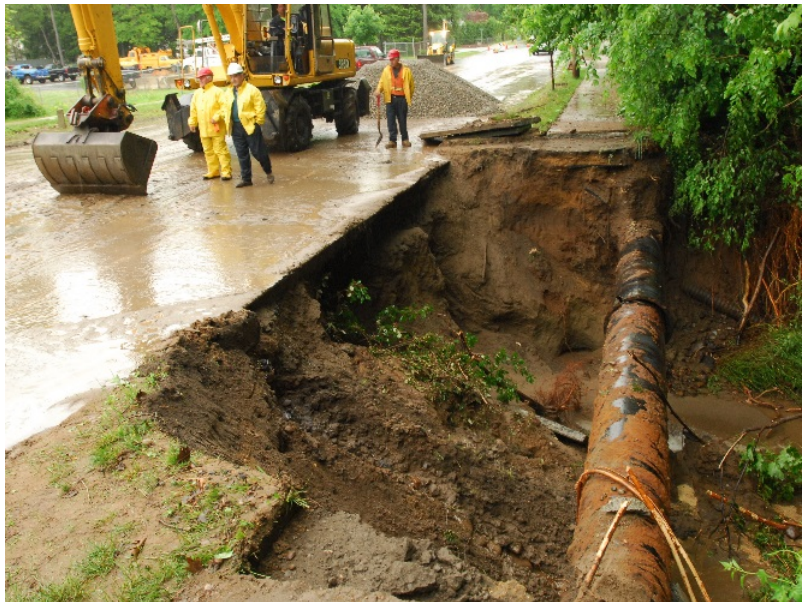
Figure 22. Fixing water main breaks is the most common direct conservation effort undertaken by Minnesota water suppliers.
