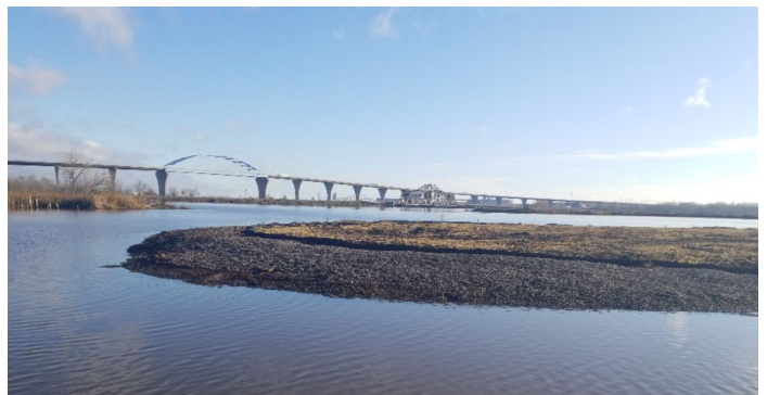
Gravel protects the new island in a high-energy area
