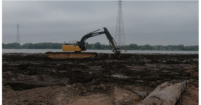
Capping the new island with clean sediment from Kingsbury Bay
