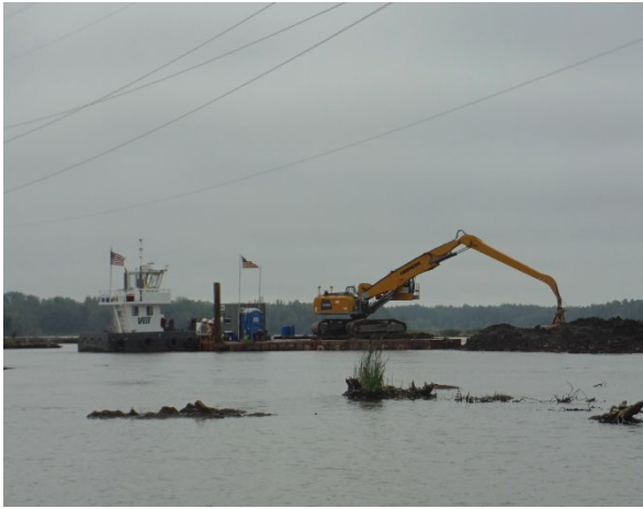
Photo Caption: Kingsbury Bay sediment is used to cap the new island at Grassy Point (left photo); after capping, the sediment is graded (right photo).
