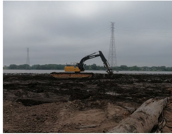
Photo Caption: Kingsbury Bay sediment is used to cap the new island at Grassy Point (left photo); after capping, the sediment is graded (right photo).
