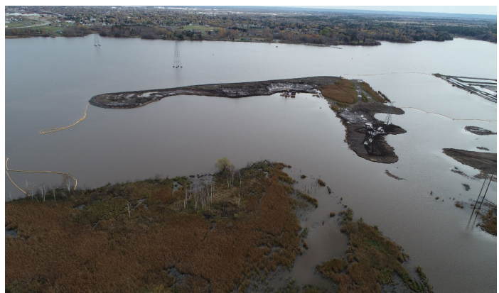
Capping the large Grassy Point island with Kingsbury Bay sediment
