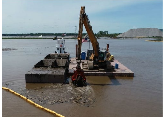
Removing legacy wood waste at Grassy Point
