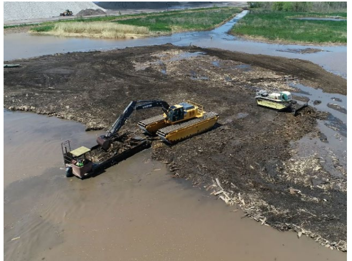
Using wood waste to construct the small Grassy Point island
