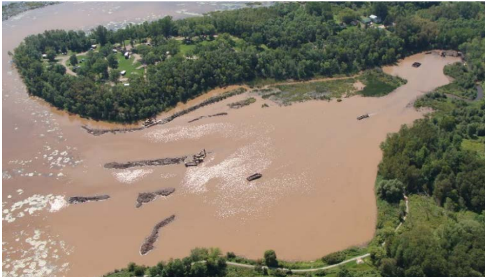
Left: amphibious excavators remove invasive plants at Kingsbury Bay;
