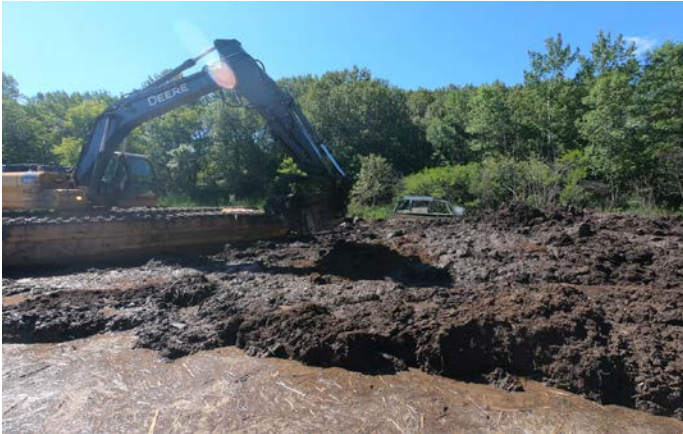
Left: an amphibious excavator removes invasive plants at Kingsbury Bay; Right: wood waste forms a new island at Grassy Point
