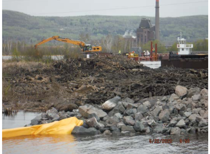
Photo: Excavating legacy wood waste at Grassy Point
