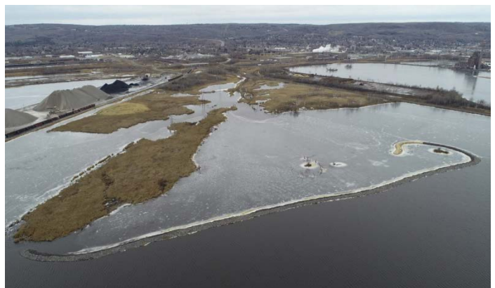
The completed berm will contain the future Grassy Point island
