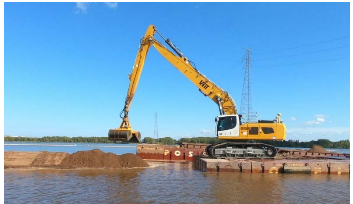
Sand is placed to form a berm at Grassy Point
