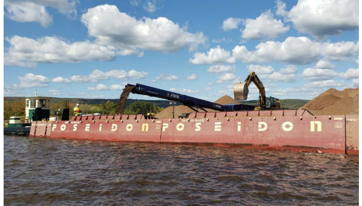
A conveyor loads sand berm material onto a barge
