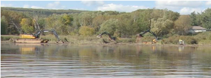
Excavators remove invasive vegetation from the Kingsbury Creek delta.
