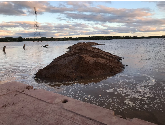
Grassy Point restoration, creation of sand berm.
