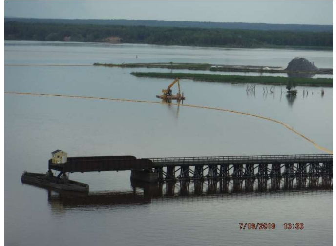
Installing Grassy Point silt curtain
