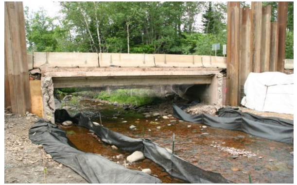
figure 4. Redundant BMPs for added protection of the waterway
