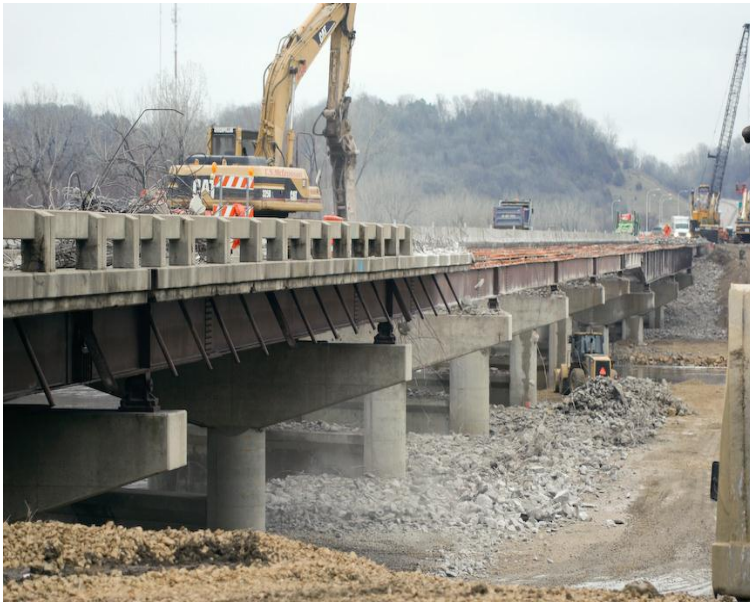
figure 1. Temporary causeway built for demolition and construction
