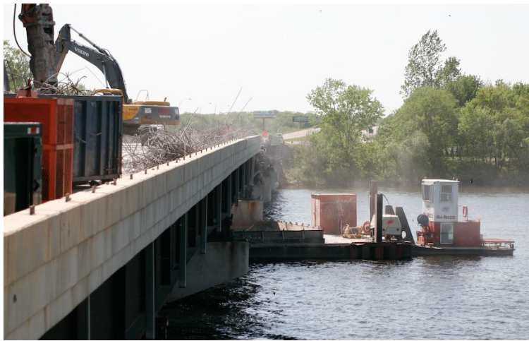
figure 2. Barge use for capturing debris
