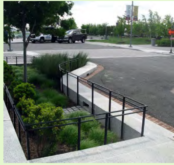
Stormwater planter boxes
