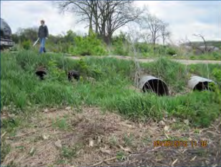
3. Floodplain Culvert Design: road bisecting the floodplain, but with floodplain culverts
