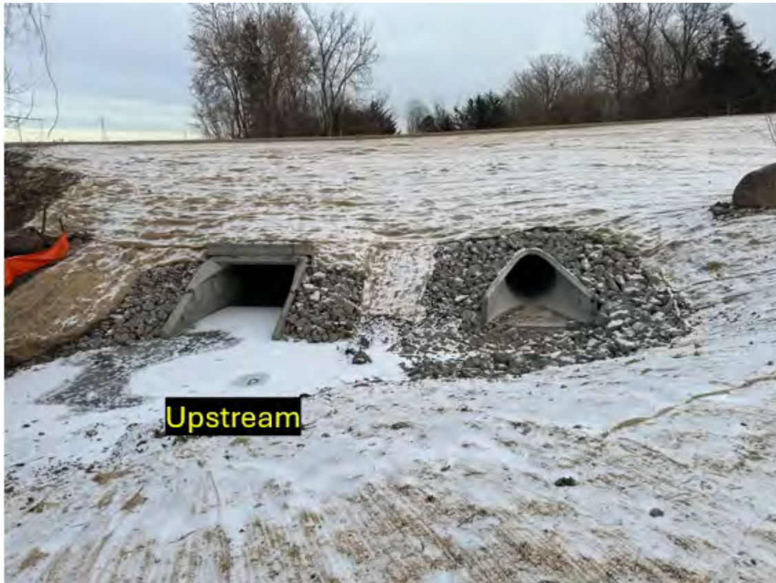
Proposed: 8 x 5 box culvert and 4-ft CMP
