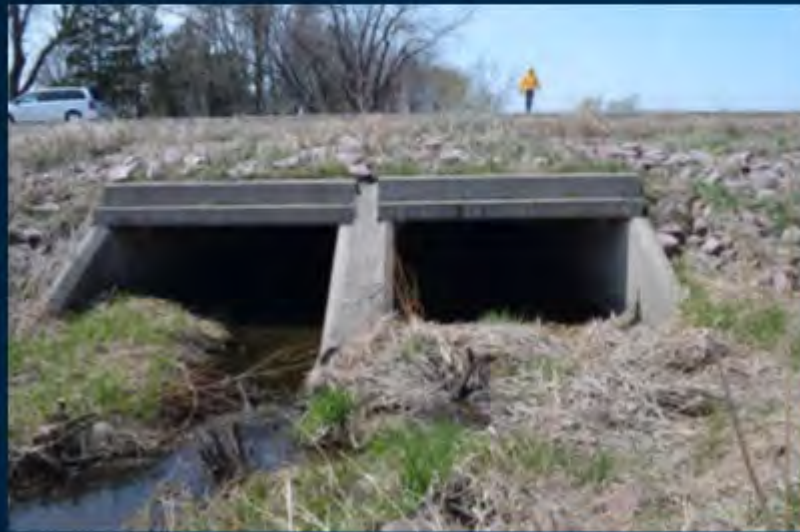
The culvert width is significantly wider than the channel width. (J. Kozarek photo).
