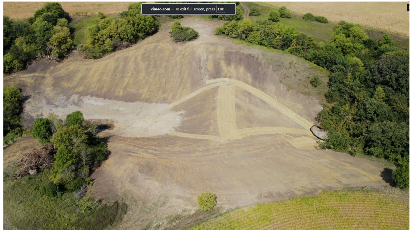
Area II Grade Stabilization Structure (drone footage from D&G Excavating)
