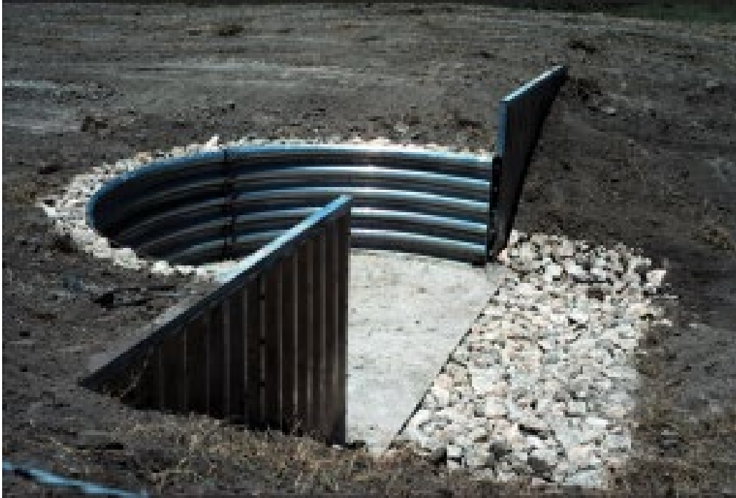
Grade Stabilization Structure (Photo from NRCS Practice Standard)
