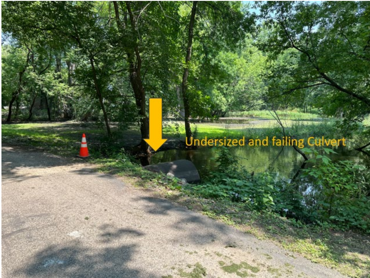
13 th Street and Mill Creek Chatham Township, Wright County
