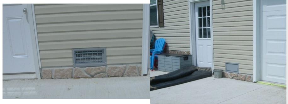
Sizing and placement of flood vents
