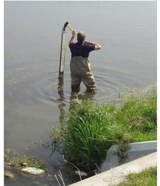
DNR staff member installs a gage in a Polk County lake.
