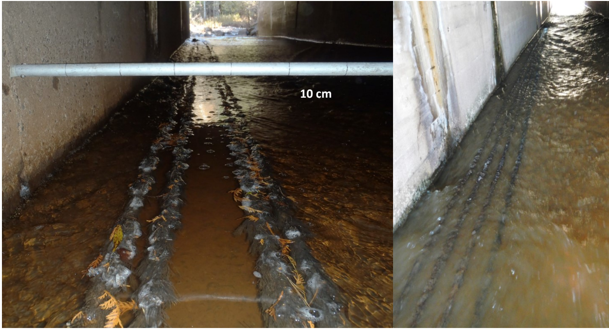
Figure 6.5.3. A recent MnDOT project explored the use of ropes originally designed for ocean mussel aquaculture as a culvert retrofit to add local roughness and cover to enhance AOP in shallow, fast flows. Still water between the sets of ropes at low flow is shown in the left image, while local reductions in velocity near the ropes slightly higher flow are evidenced by variation in surface flow patterns at right. Both photos are looking upstream. Photos M. Hernick and R. Gabrielson (2017).
