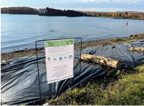
Figure 3: In process picture of Agate Bay restoration 09/2024
