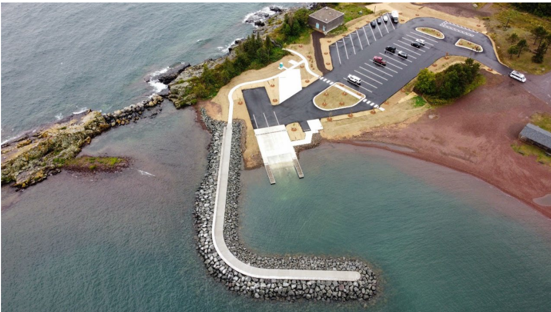
Photo 1 caption: Aerial view of the breakwall and parking lot at the public access site in Grand Marais, with stormwater amenities completed.
