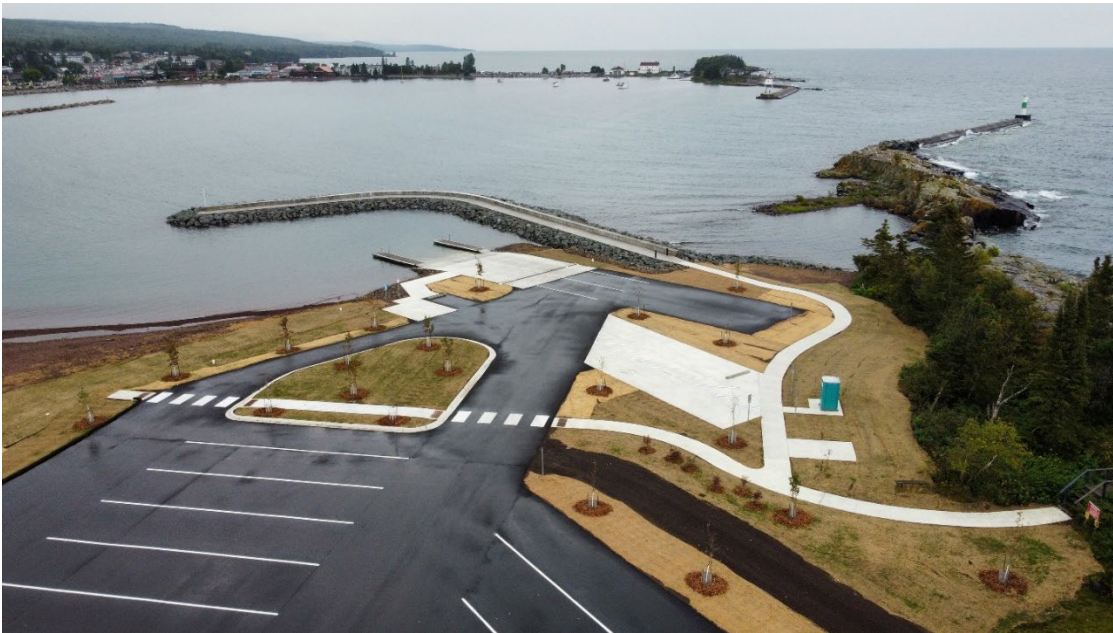
Photo 2 caption: (closer) Aerial view of the breakwall and parking lot at the public access site in Grand Marais, with locations of stormwater amenities such as trees.
