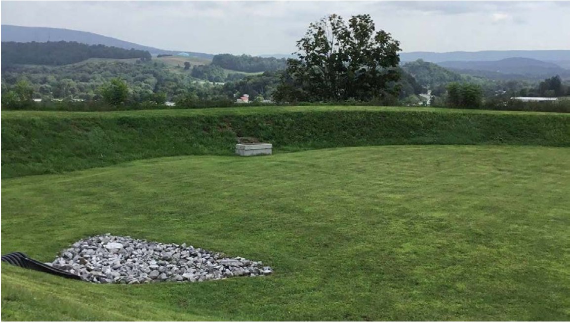
Image 5: Infiltration Basin Photo
