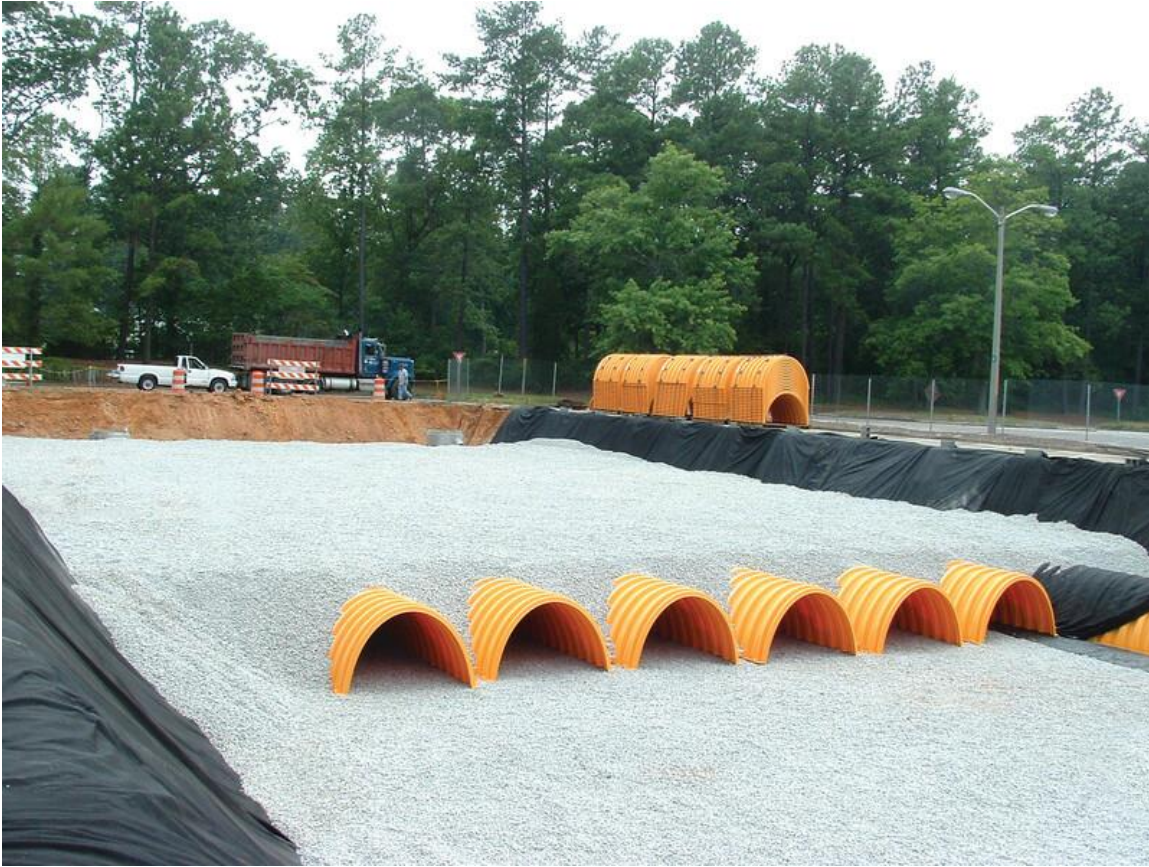
Image 2: Subsurface Drain field During Construction
