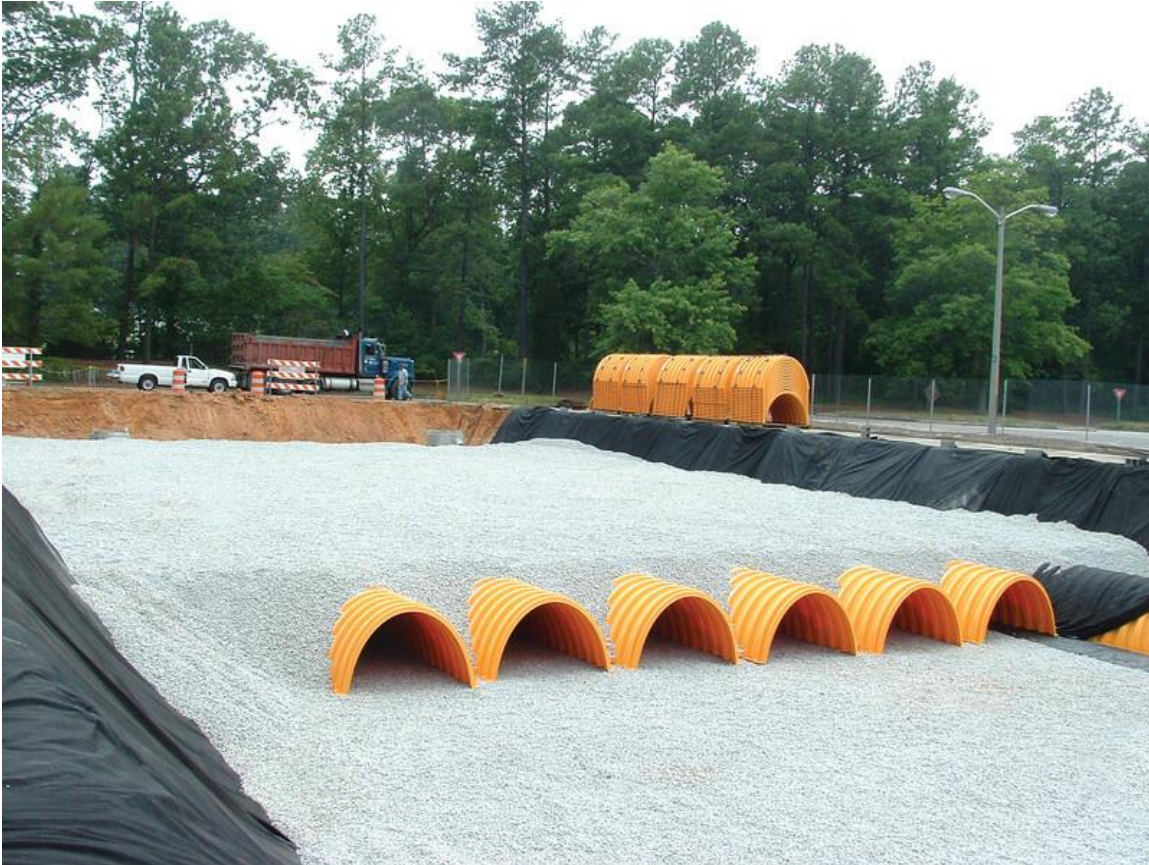
Image 2: Subsurface Drain field During Construction
