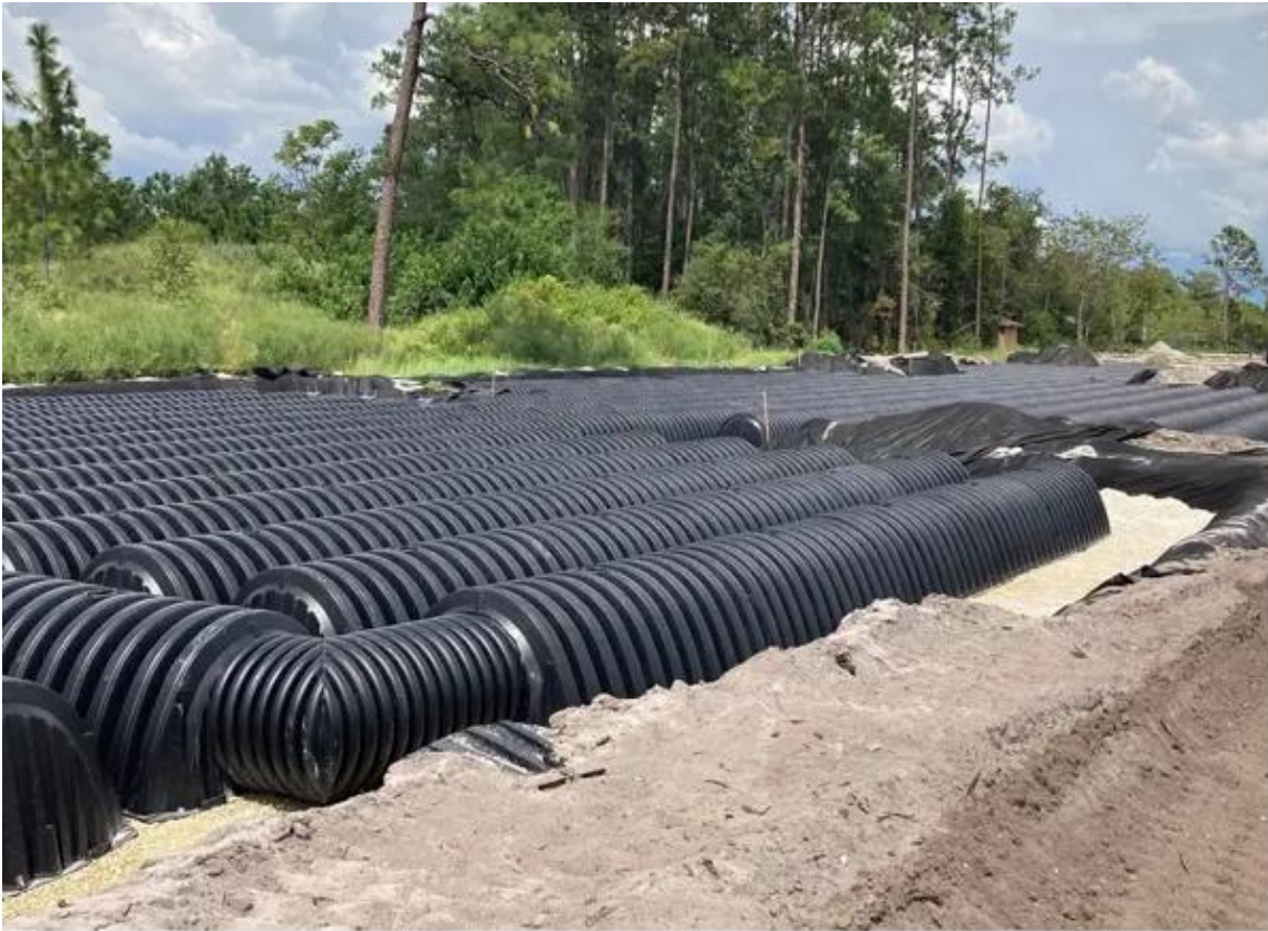
Image 1: Subsurface Drain field During Construction
