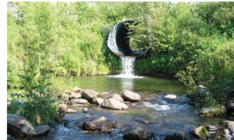
Dams and culverts: (above) A handmade dam disconnects fish from upstream migration and alters the streamflow. (below) A perched culvert also inhibits fish passage and disrupts the longitudinal connectivity of the stream.
