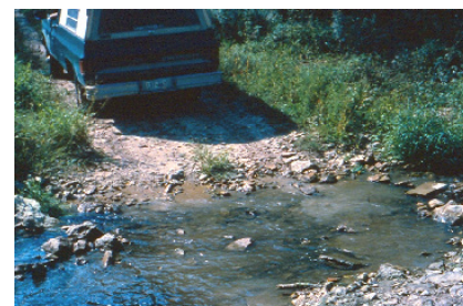
A low-water ford crossing is designed for infrequent use by vehicles.
