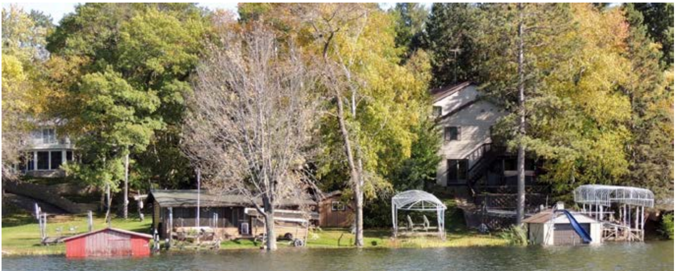
Flood prone accessory structures on a lake with fluctuating water levels. Photo credit: Lake Shamineau Lake Improvement District
