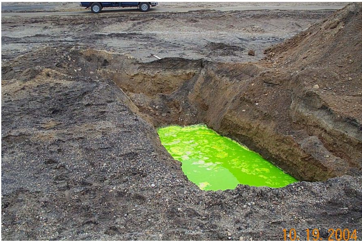
Figure 8.6. Trench 1, dye injection point.
