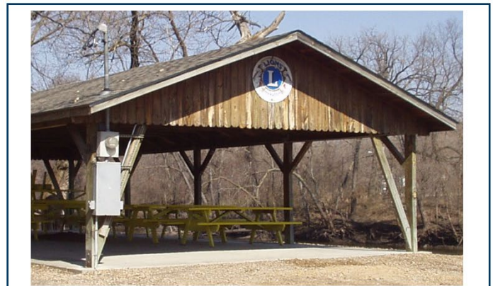
Figure 4. An open-sided picnic shelter with slab on grade foundation anchoring may be below the RFPE if flood-resistant materials are used. Note the elevated utilities.
