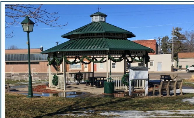
Figure 3. A gazebo with a roof but no solid walls may be below the RFPE if adequately anchored and constructed using flood-damage resistant materials.
