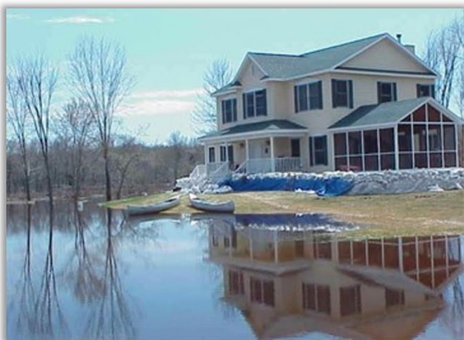
Figure 1. A properly elevated residential building in the flood fringe.
