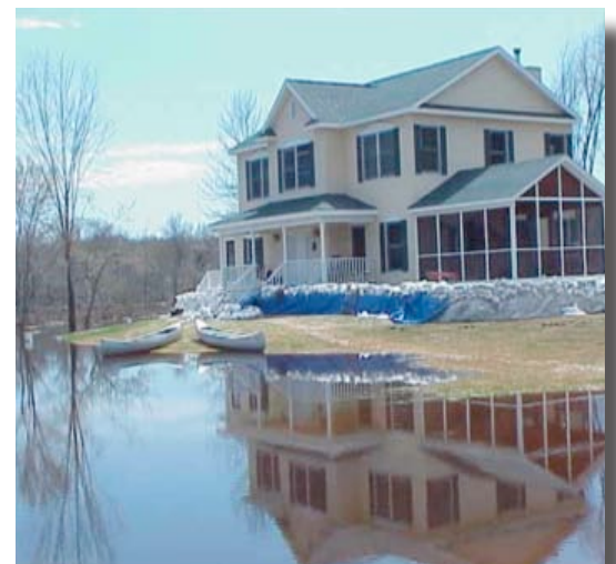
Figure 1. Houses may be constructed in the flood fringe but must be properly elevated to maintain public safety and minimize damage risk during a flood.
