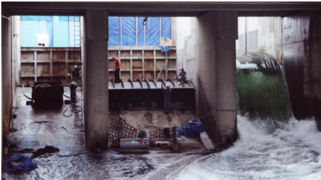
Start of Installation – Installing Gate Panel – Completed Gate
