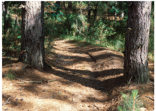
Although this OHM trail is in sandy, noncohesive soil, systematic displacement on the curve has formed a superelevated curve that limits further displacement. Since the tread remains porous and the site has only gentle slopes, erosion is not a problem and trail is sustainable.
