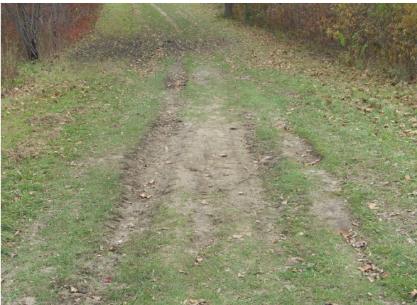
Problem: Lack of underlying soil stability. Organic soils are inherently prone to rutting. Although still within rutting limits, this trail is close to becoming unsustainable, especially if soils begin to migrate to adjacent systems and water bodies. If foot traffic is low, periodic reseeded and filling may be the best approach. If the problem continues, rerouting may be necessary.
