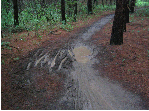
Problem: Trail creep. This low spot on a mountain bike trail is routinely wet, forcing trail users to go around it. Either a reroute or hardening with rocks or a boardwalk is necessary to avoid continued expansion of the trail.
