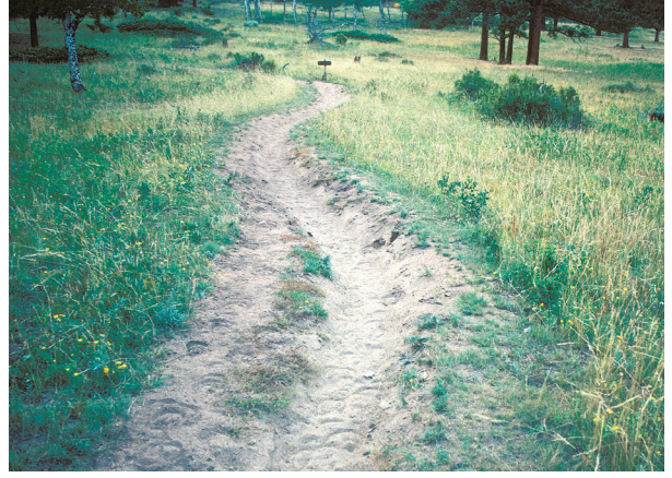
Problem: Soil limitations. With sandy soils, trail creep can become a sustainability issue. If this is limited to an occasional stretch, no major action is required. But if this problem persists over a significant distance, rerouting or closure may be necessary.
