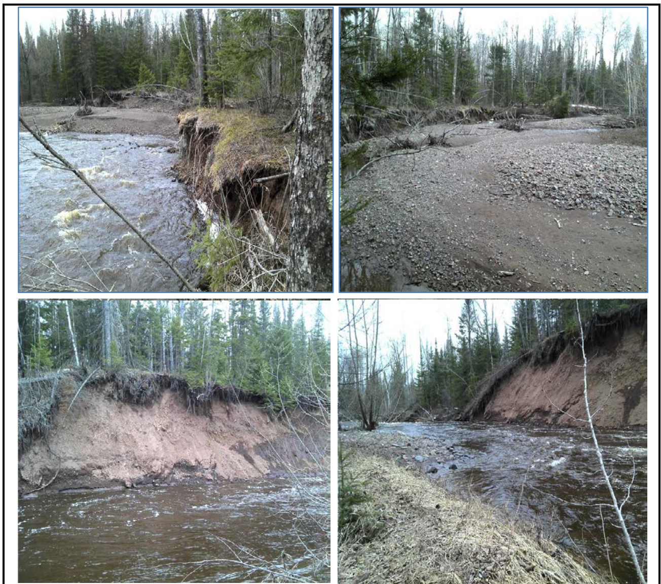
FIGURE 11. Proposed stream restoration area by Lake County SWCD on newly acquired Stewart River easement.
