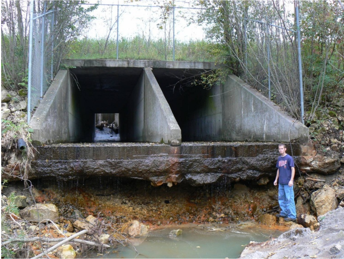
Figure 6. Improperly designed or placed box culverts at road crossings can result in barriers to fish movement, and loss of connectivity in riverine systems.
