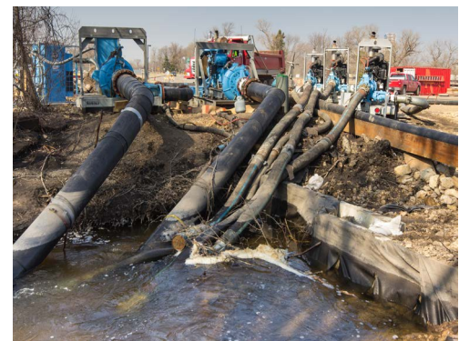
Figure 6. Drain all water from equipment where water may be trapped. Remove drain plugs and drain hoses prior to transport. Photo Credit: Peter Leete, DNR
