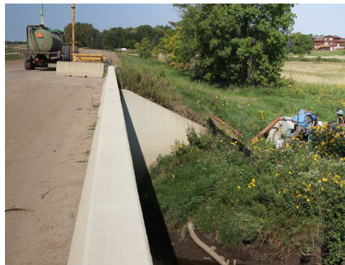
Figure 5. Pumping from designated infested waters for use elsewhere on the project is prohibited without a permit. Photo credit: Peter Leete, DNR
