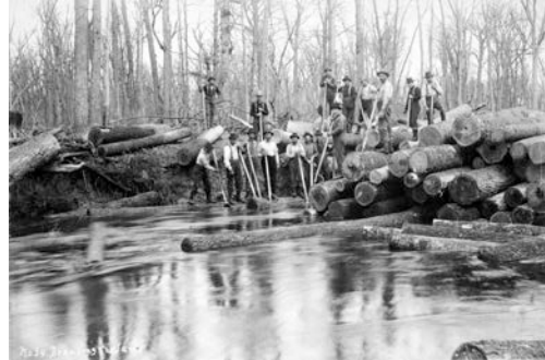
Figure 3. Log drivers moving timber, bundled in “pigs”, downstream.
