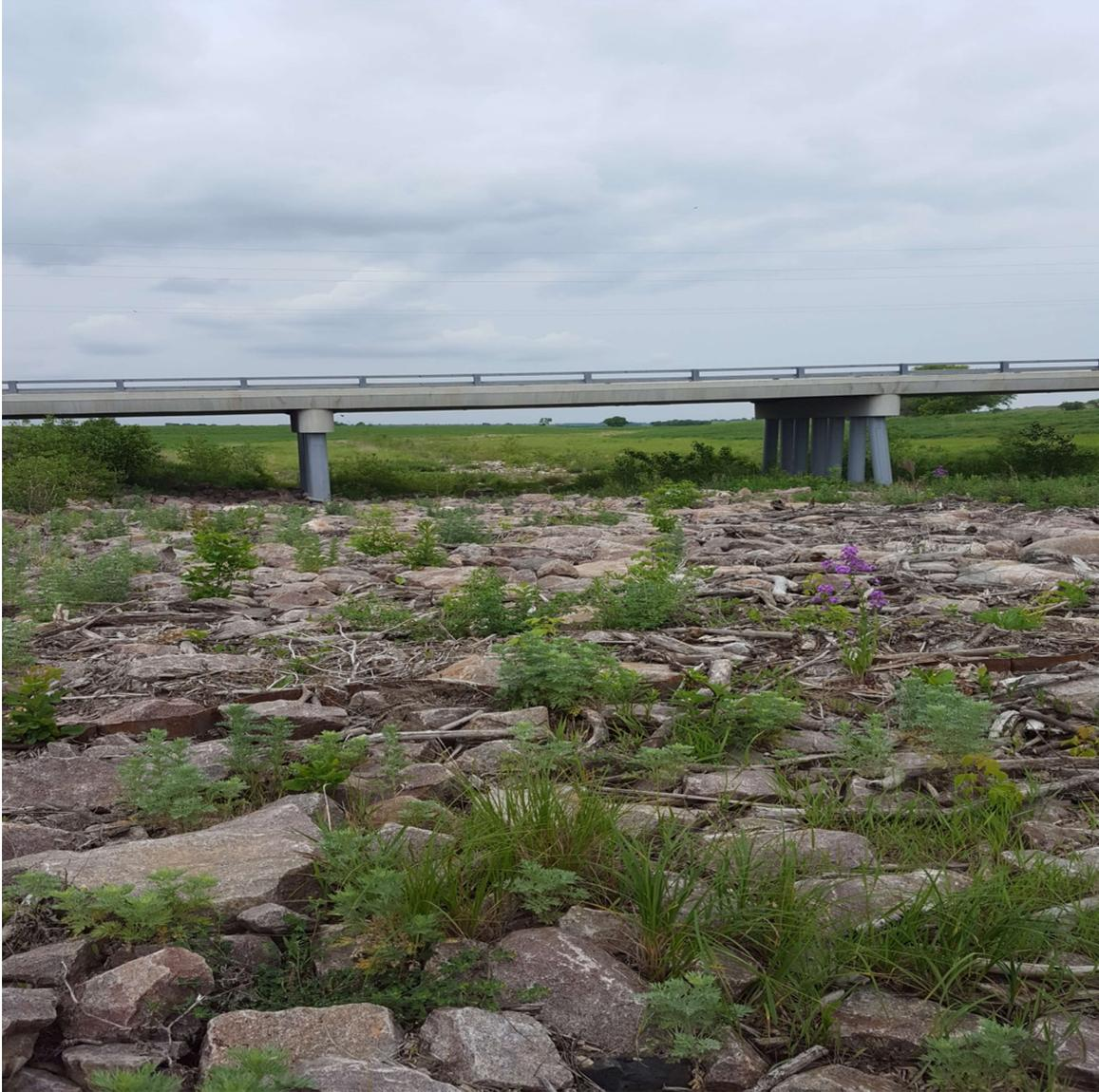
**Picture 3.** The structure Houston Engineering built to relieve flooding. This allows water to flow to a downstream part of the Little Minnesota River (below Browns Valley). The rocks are put there to stop scour around the bridge and elevate the side channel to allow it to be only used when an ice jam occurs.
