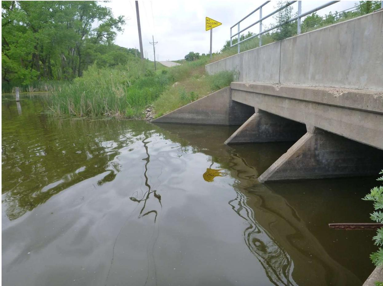
**Picture 5.** This is the box culvert leading from the Lake Traverse to the south side of the highway. The box culvert is always open and does not have a gate to stop flow, so when the Little Minnesota River floods into Lake Traverse the water does not have any restrictions to prevent connecting the two watersheds.
