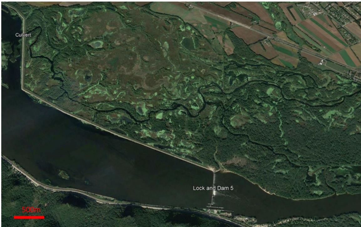
Figure 49: Map of Lock and Dam 5 showing the location of the culvert to the northwest.
