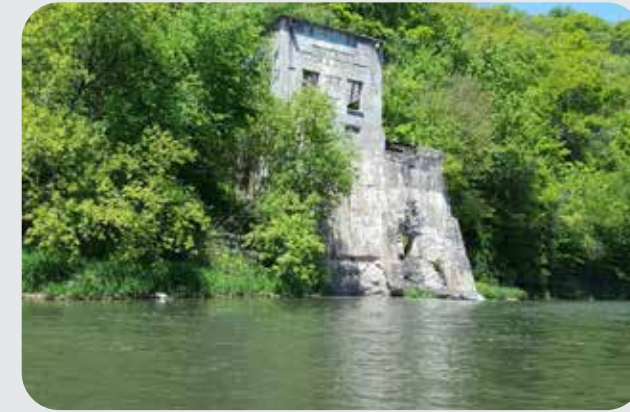
An old power station is a fun sight along the river.
