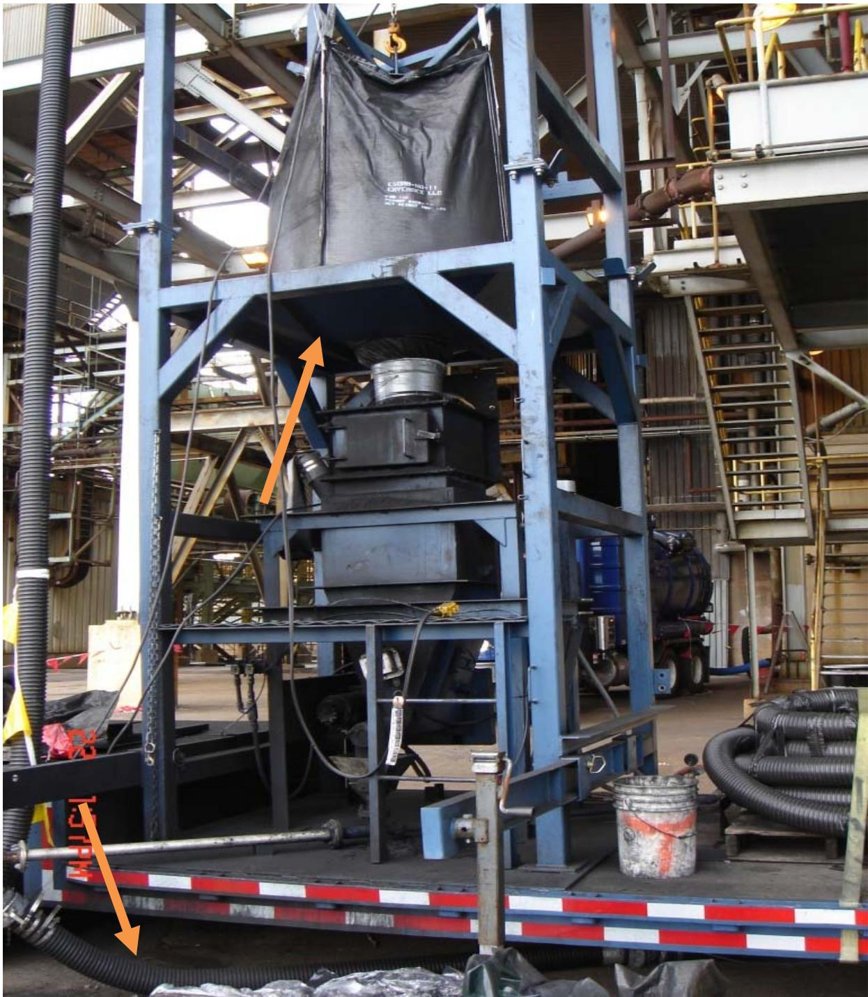
Figure 1. A close-up photo of the sorbent bulk-bag handling system. The bulk bag is placed on the top (upper arrow). The discharge pipe below (lower arrow) comes from the educator and is attached to a hose that connects to the distributors and injection lances.
