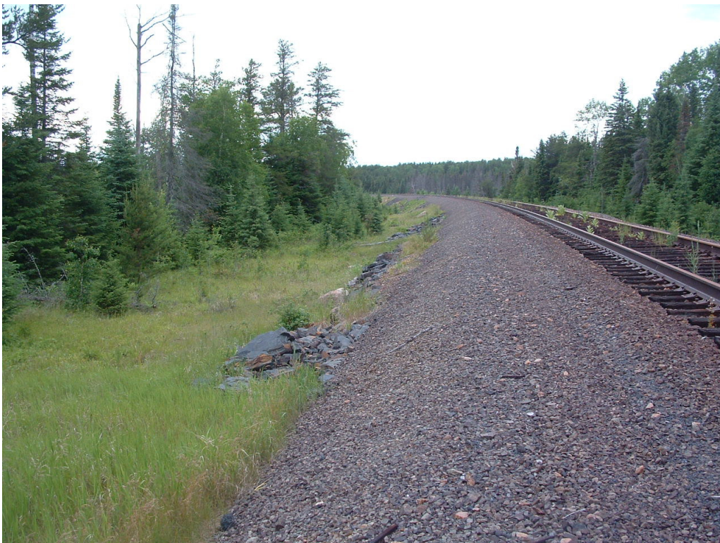
Photo 12. Polymet 18, railroad right-of-way (looking east).
