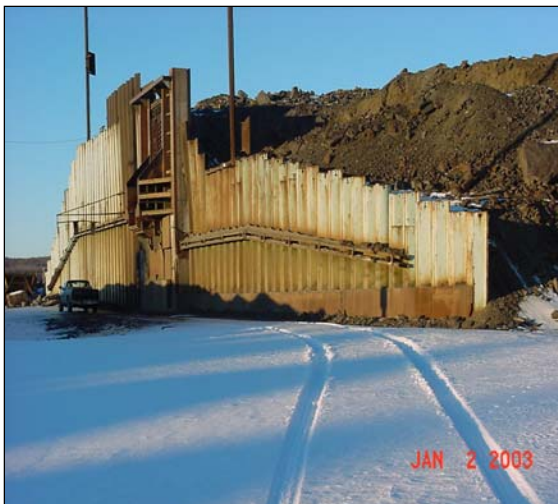
Figure 9. Mechanized loading pocket used to load rock onto rail cars.
