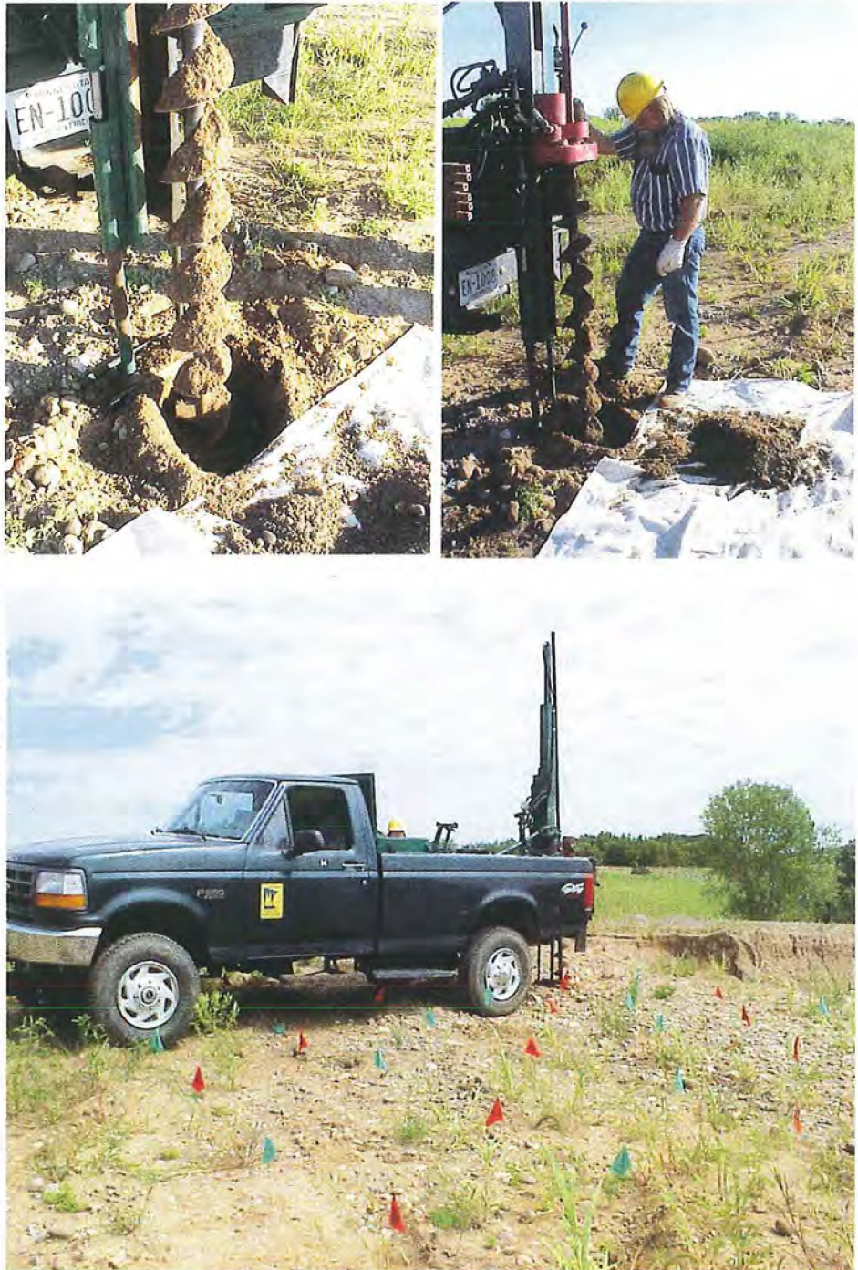
Figure 4. A Giddings Soil Probe was used for the testing. The different diameter auger flights are interchangeable on this machine.
