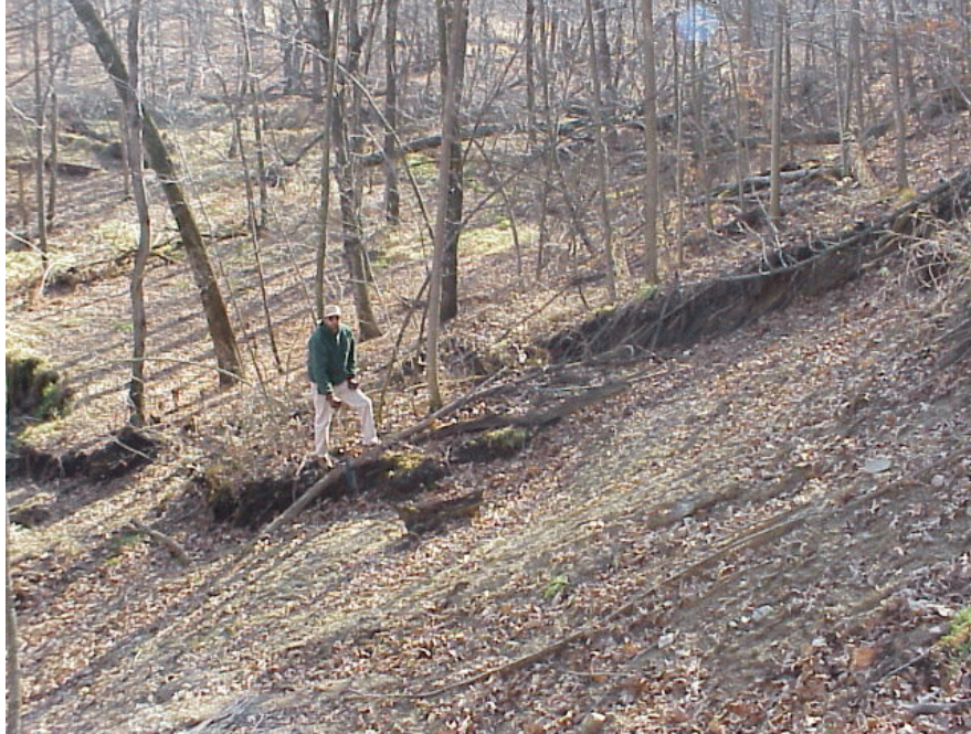
Figure 5. This slope failure occurred when this mass of vegetation and soil slid about 20 feet down this slope sometime in the last several years. The stream is just off the left side of the photo.
