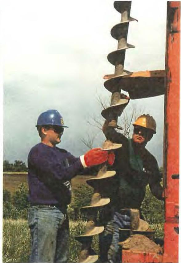
Figure 4. Five foot auger sections were added to the 25 ft auger to reach thicknesses of over 50 feet (right).
