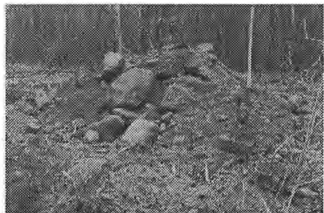
Figure 5. Spoil pile from backhoe excavation. Note the numerous relatively large boulders present. Length of shovel handle is 3.25 feet.
