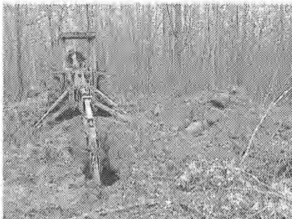
Figure 4. Backhoe excavating trench in preparation for drilling.
