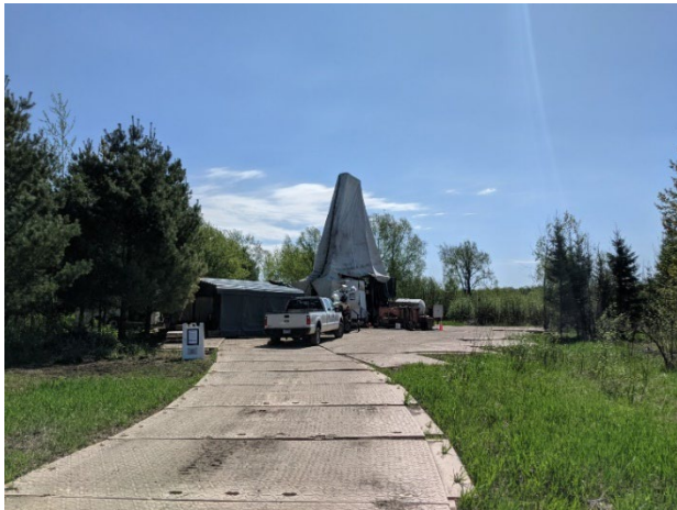
Drill Site May 2022 – note the use of composite mats that minimize soil disturbance.
