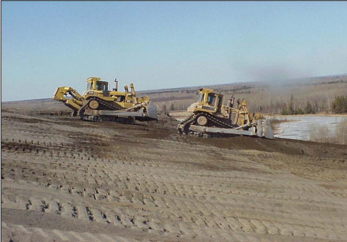
Figure 2. Coarse tailings dike being sloped at United Tac prior to reclamation.
