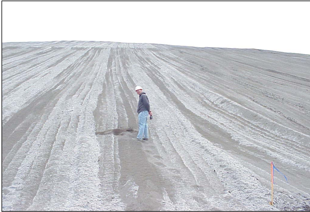
Figures 14 and 15. Before and after seeding of the 2002 demonstration plots at United Tac tailings dike utilizing WLSSD anaerobically digested biosolids mixed with Stora Enso paper waste. The small bin plots can be seen in the picture below.
