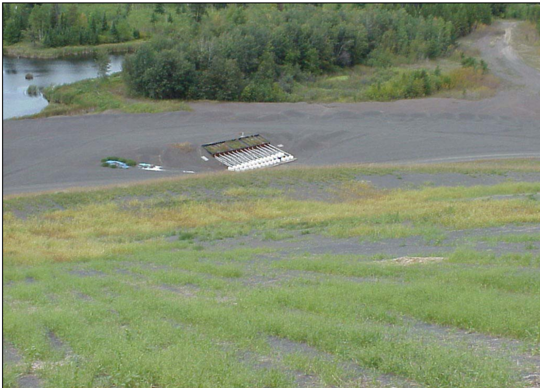
Figures 14 and 15. Before and after seeding of the 2002 demonstration plots at United Tac tailings dike utilizing WLSSD anaerobically digested biosolids mixed with Stora Enso paper waste. The small bin plots can be seen in the picture below.
