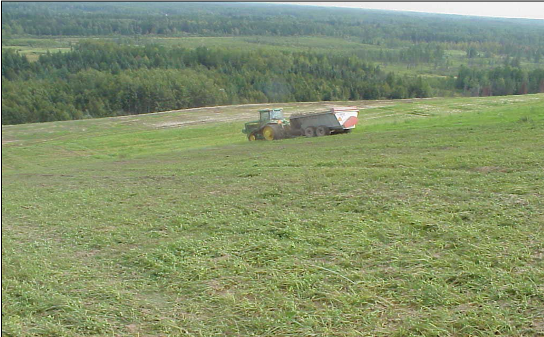
Figure 4. Western Lake Superior Sanitary District (WLSSD) biosolids being surfaced-applied to existing vegetation on a slope at the United Taconite tailings basin.
