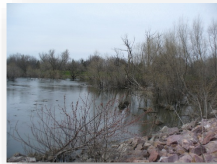
Floodwaters viewed from Dynamite County Park, River Road
