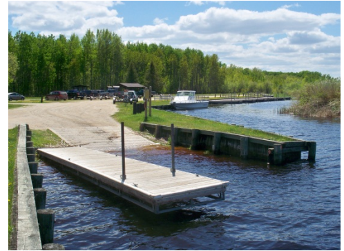
The existing harbor in Zippel Bay was rehabilitated in 2014 to replace the seawall, dredge the harbor, increase docking capacity and improve the boat ramp. Additional improvements will be planned.
