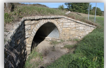
WPA-constructed culvert in the new campground area
